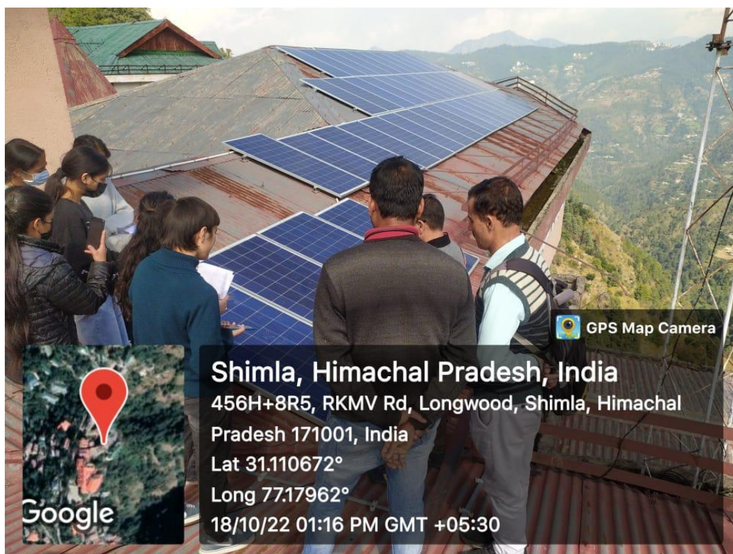
Rooftop Solar Power System Installation in Science Block
